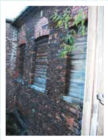
Details of the original building are still visible
